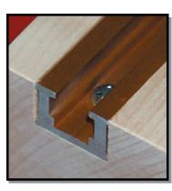
Build-up Use 1/2" thick material on either side of a surfacemounted track to create a flush mount.
